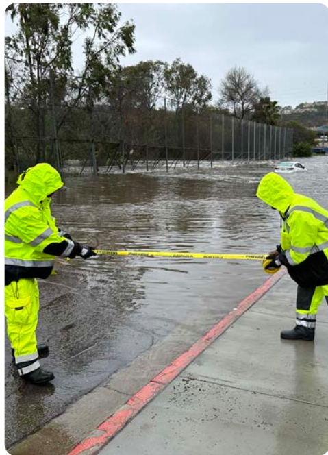
Stormwater crews respond during storms where flooding issues are reported.
