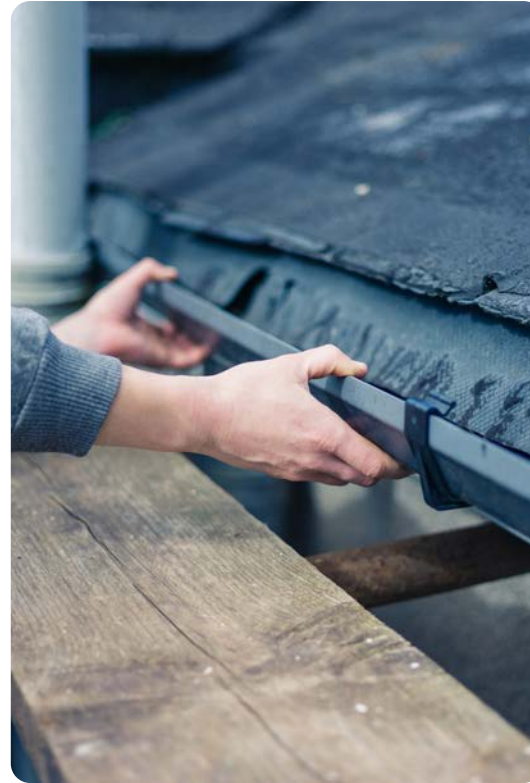
Rain Gutter Replacements
