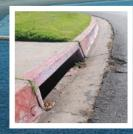
Storm drains collect rain water to help prevent flooding in our communities. The storm drain system includes a vast network of underground pipes and open channels that take water away from streets and other developed areas. Water <u>enters</u>
