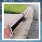
Storm drains collect rain water to help prevent flooding in our communities. The storm drain system includes a vast network of underground pipes and open channels that take water away from streets and other developed areas. Water enters
